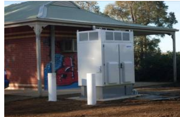
5 kW ElectraGen™XTi Fixed/BTS Broadband site Victoria (Australia)
