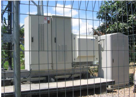
2.5 kW ElectraGen™H2 BTS (Indonesia)
