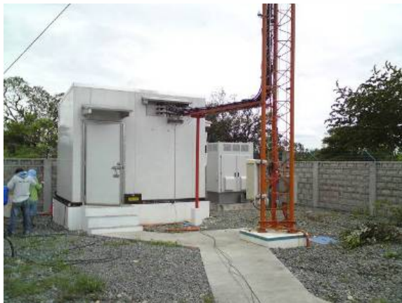
5 kW ElectraGen™XTi BTS (Philippines)
