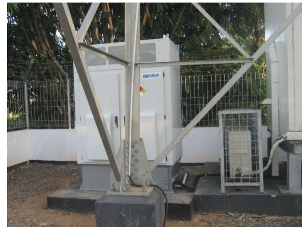
3 kW ElectraGen™XTi BTS (Indonesia)
