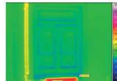
2b: Thermographic image
